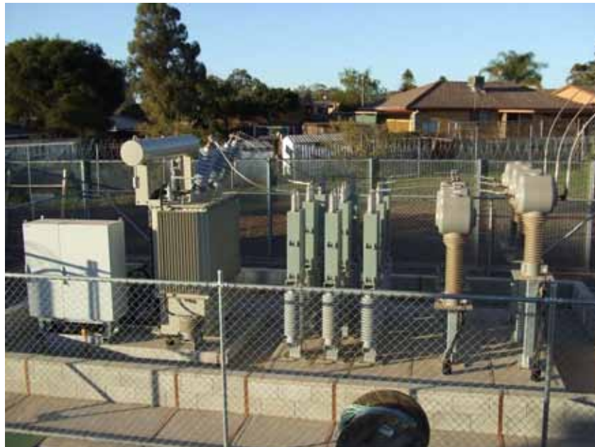
Figure 3.3: Ripple Injection Equipment at a Zone Substation (photograph courtesy of Essential Energy)
